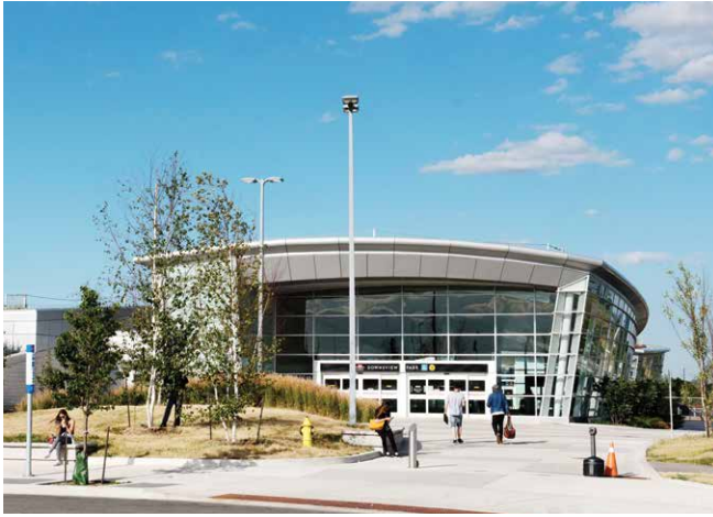
Downsview Park Subway Station
