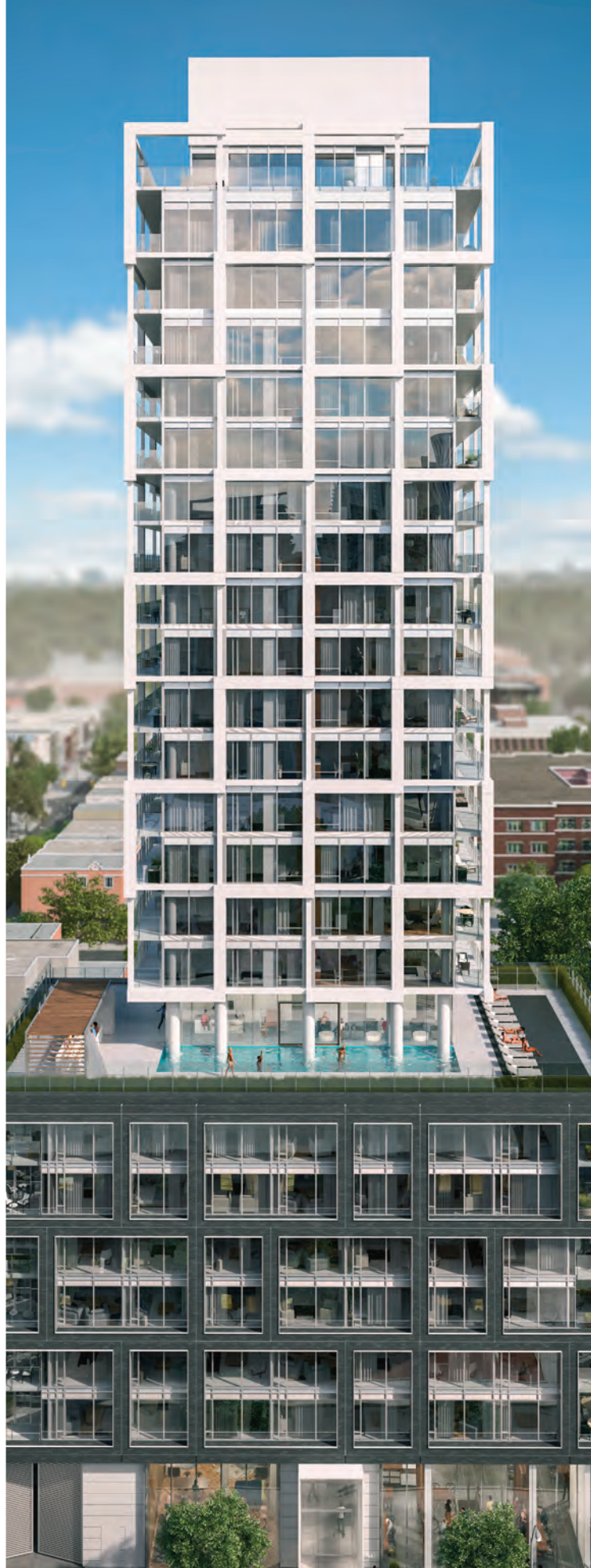
EAST FIFTY FIVE, TORONTO UNDER CONSTRUCTION
