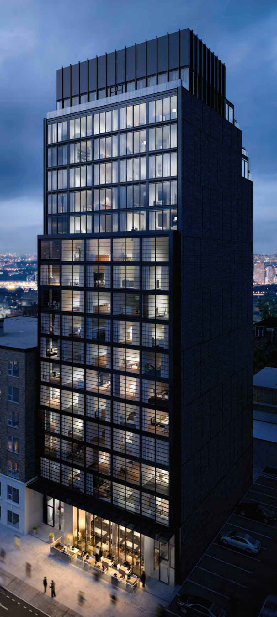
WOODSWORTH, TORONTO UNDER CONSTRUCTION
