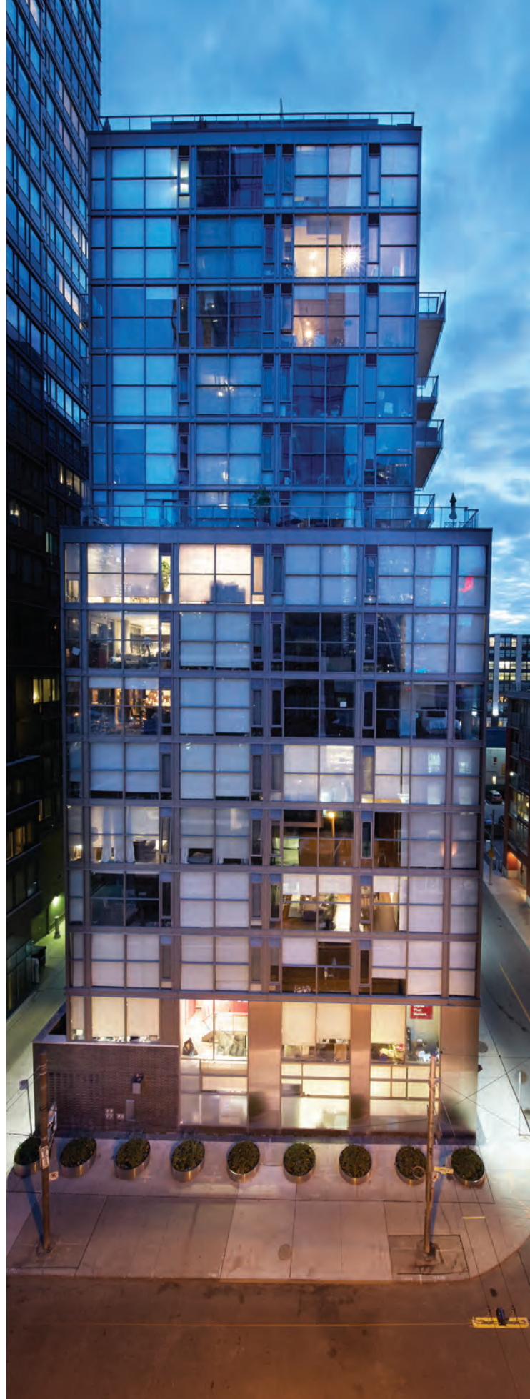
GLÄS, TORONTO COMPLETED 2009
