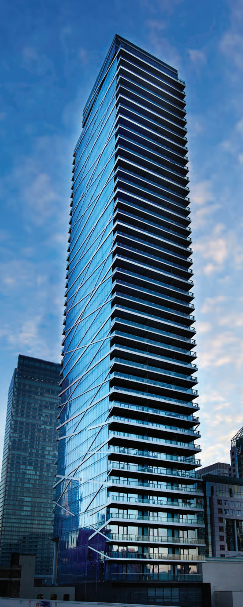
THEATRE PARK, TORONTO COMPLETED WINTER 2014
