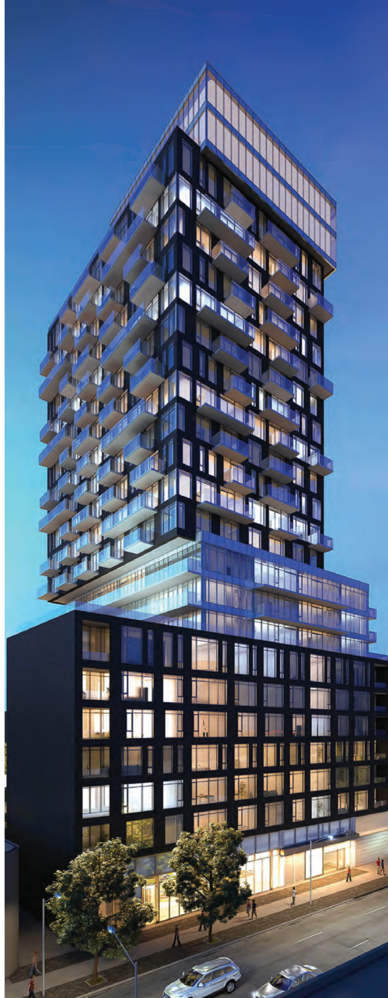
SOBA, OTTAWA UNDER CONSTRUCTION
