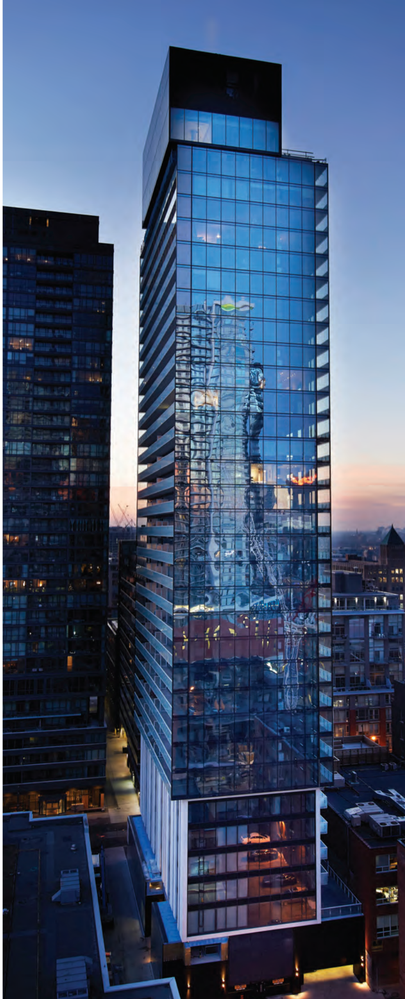
KING CHARLOTTE, TORONTO COMPLETED FALL 2015
