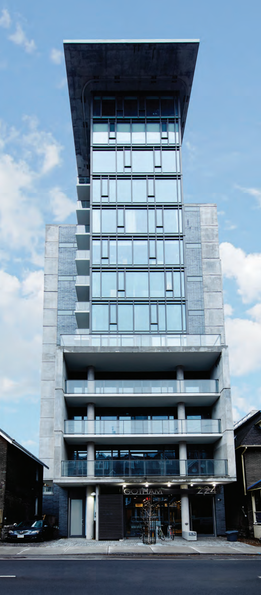
GOTHAM, OTTAWA COMPLETED SPRING 2015
