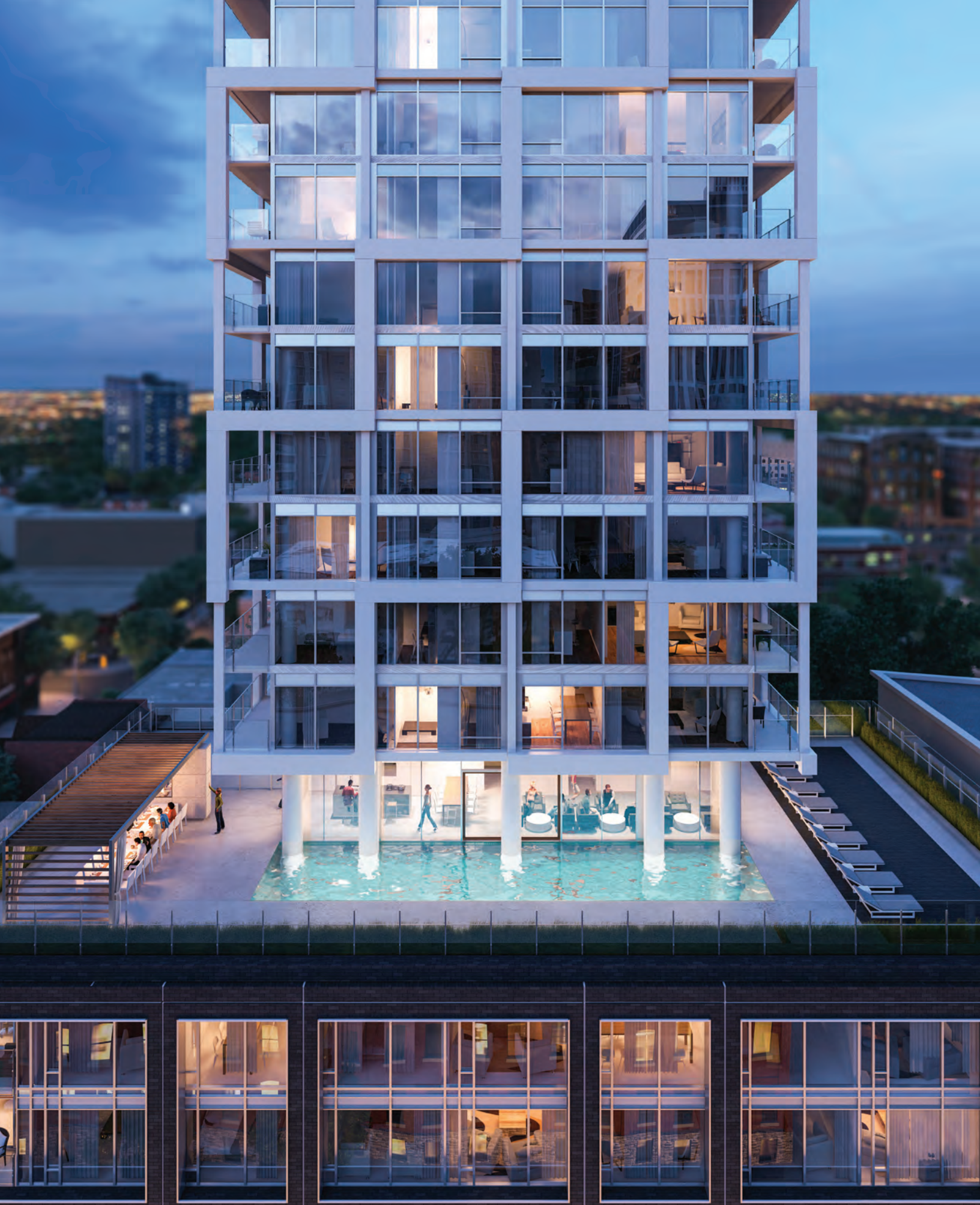
EAST FIFTY FIVE, TORONTO UNDER CONSTRUCTION
